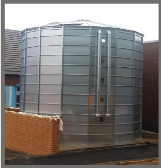
Fill & Vent Pipework – Can be supplied to allow blown deliveries of wood chip or wood pellet.
