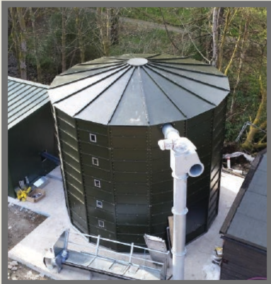
Powder Coating – Silo powder coated to match its surroundings.
